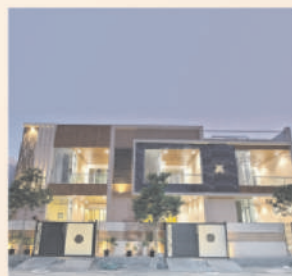
ENERGIA VILLAS Tonk Road, Jaipur
